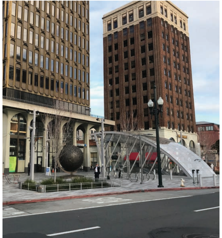
Example implementation of how a transit facility can have a seamless integration with a plaza-like area. - Photo: Community Design + Architecture
