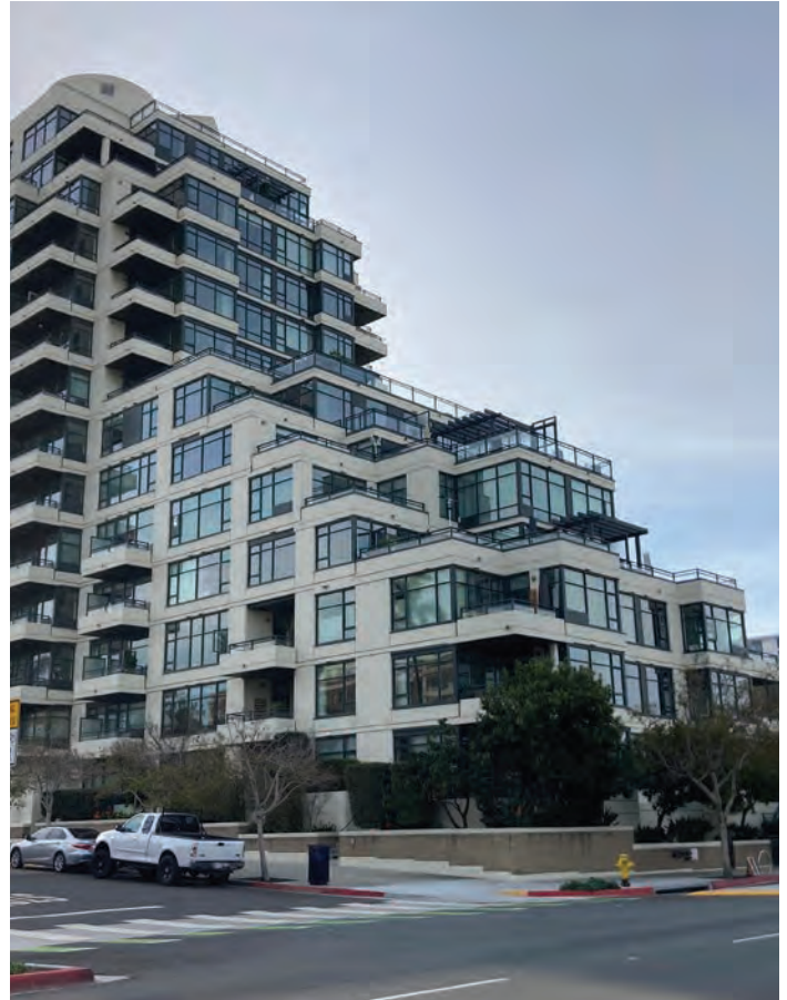
Example of a building designed to step down to reflect the site context.
