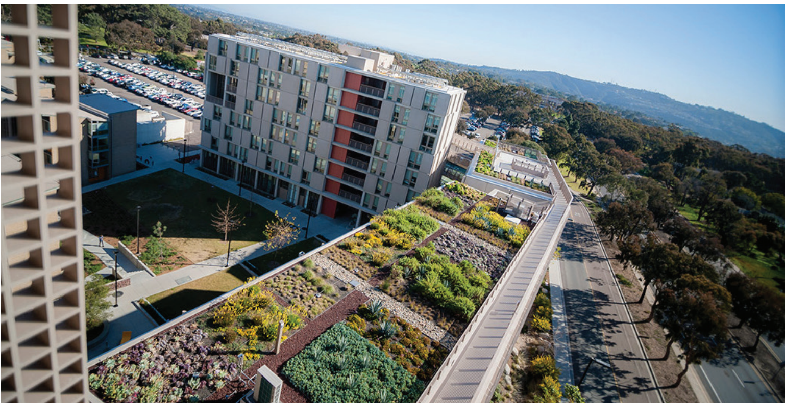
Green roof implemented at the Keeling Apartments. - Source: UC San Diego Publications
