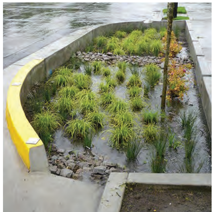
Green infrastructure like stormwater detention basins help mitigate stormwater runoff and flooding.
