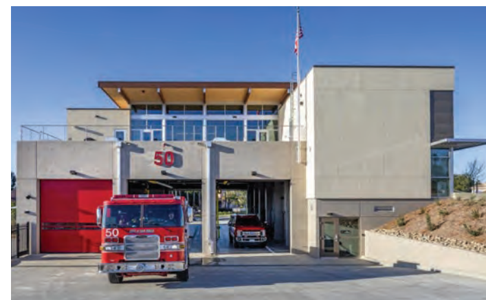
Station 50 provides fire and rescue services to the southern area of the University Community.
