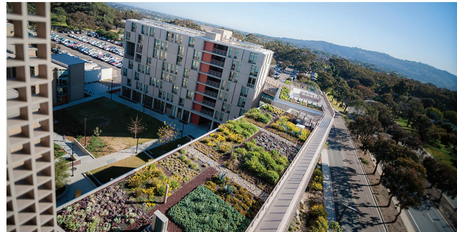
Green roof implemented at the Keeling Apartments. - Source: UC San Diego Publications
